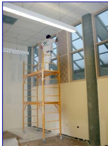
Room 1170 Remodel MacMillan Hall
