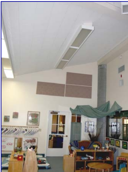
Child Development Center New acoustical ceiling tiles installed for noise reduction
